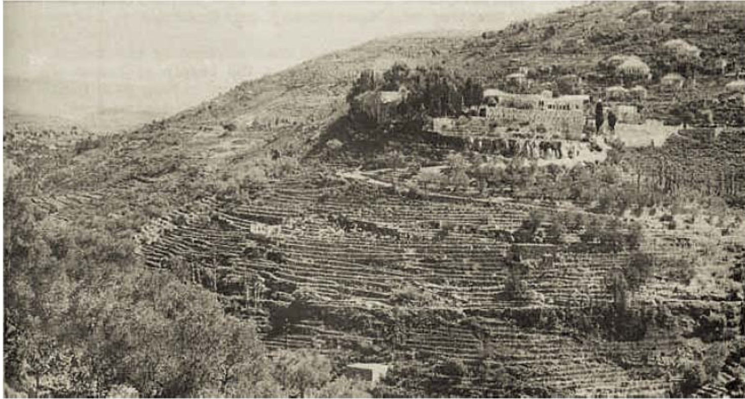
Fig. 6. Ancient rock-walled bench terraces protect this Lebanon hillside after thousands of years of use. It is estimated that the terracing of some Lebanon hillsides cost at least $2,000 per acre, if we should figure the cost of labor at 40 cents per hour. Such expensive methods of protecting the land are practical only where people have no other land on which to produce their food.
